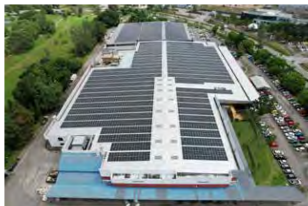
Completion of 2.5783 MWp Rooftop Solar Installation
