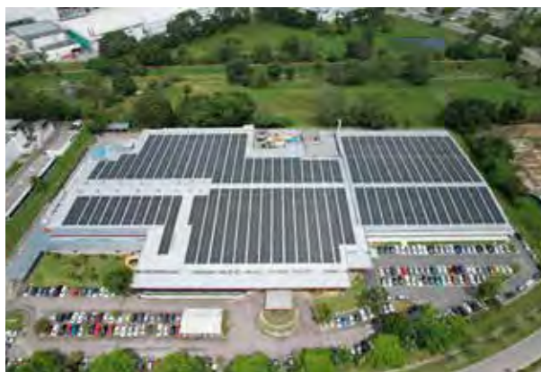
Completion of 2.5783 MWp Rooftop Solar Installation
